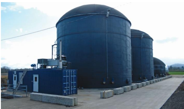
Figure 1. An anaerobic digester operating on an Oregon dairy farm. (Photo credit: Dan Sullivan) 3 .
